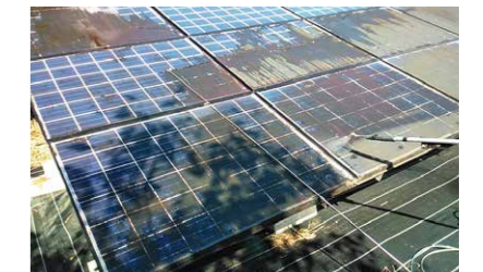
Cleaning the panel
