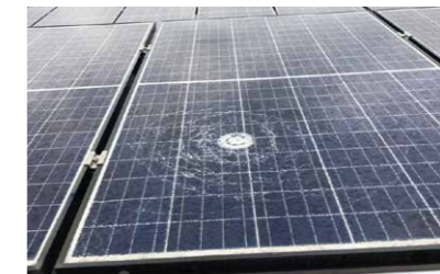
Panel damage due to falling objects
