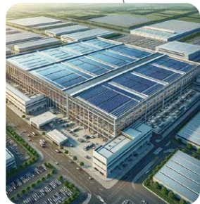
In-house power generation at corporate offices to increase productivity.
